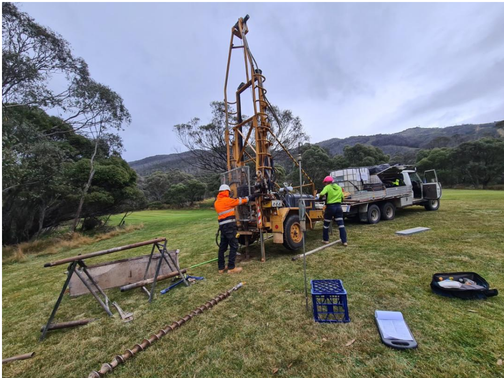
Photo 5 - Drilling and DCP Test Set Up at Borehole BH05 Looking Southwest
